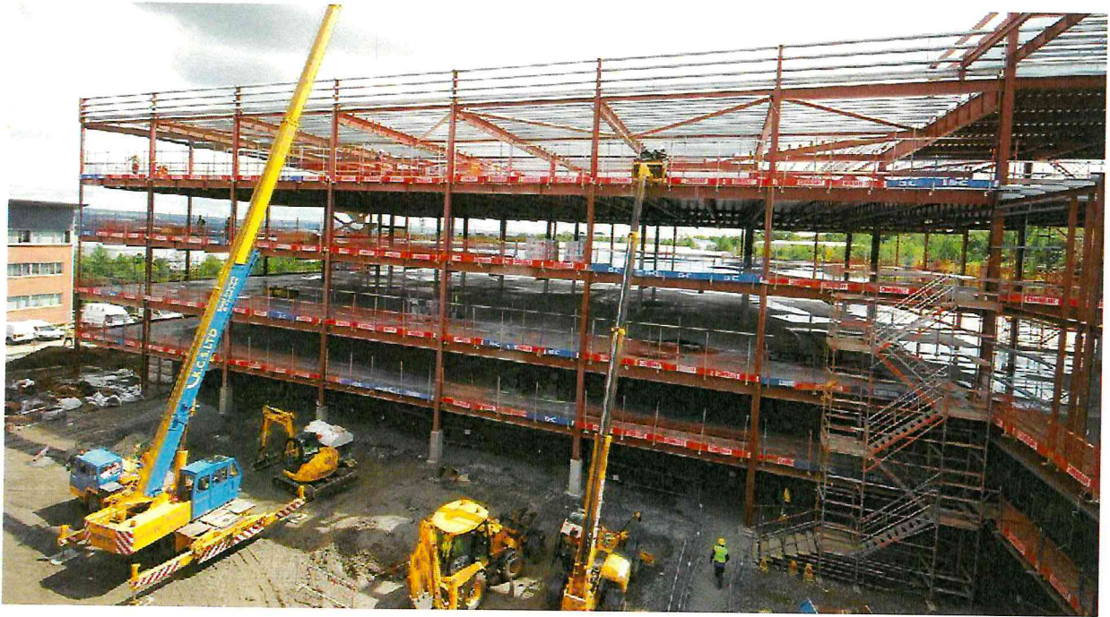
Safe means of access to, and egress from, high-level places of work should be provided
