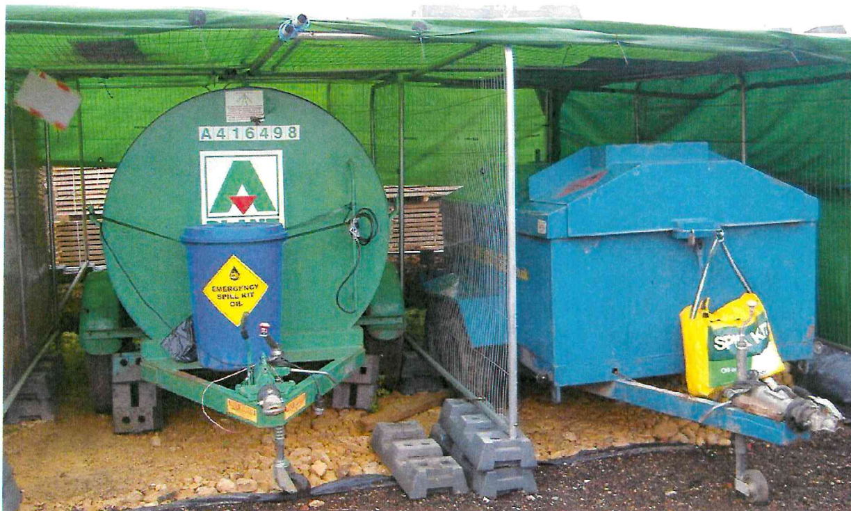
Examples of covered storage for oil
