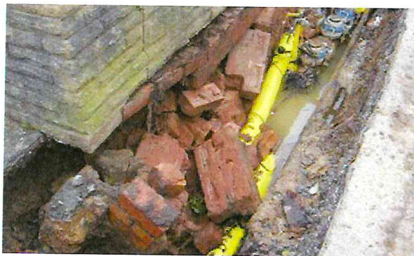
An unsupported excavation resulting in collapse
