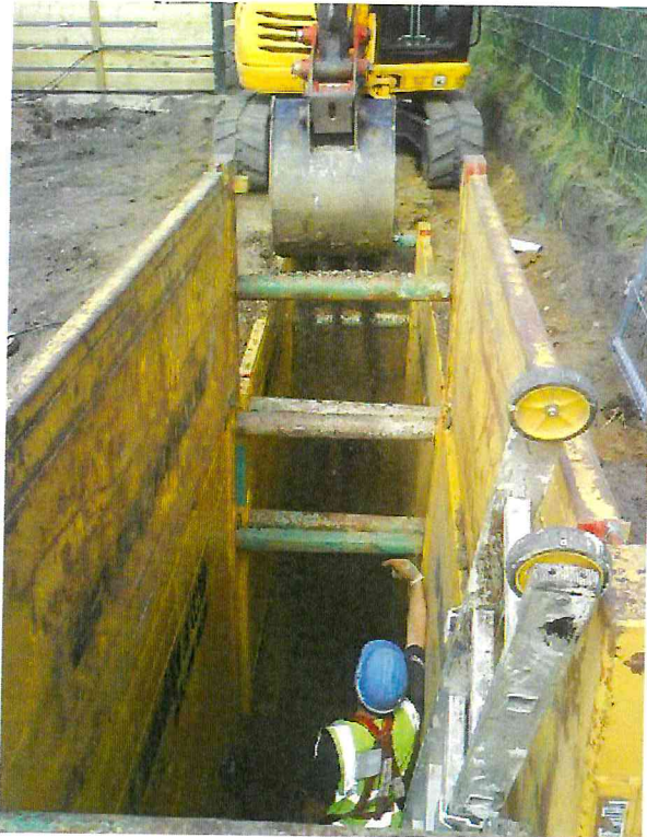
Safe working in a deep excavation using trench boxes and a secured ladder
