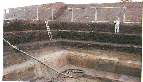
Examples of stepped excavations
