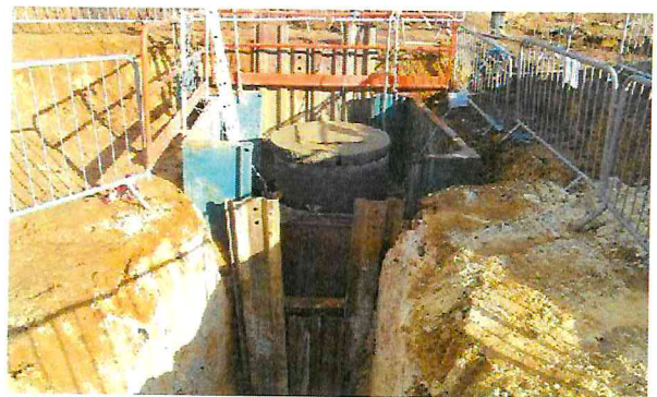
Deep inspection chamber excavation with access and edge protection
