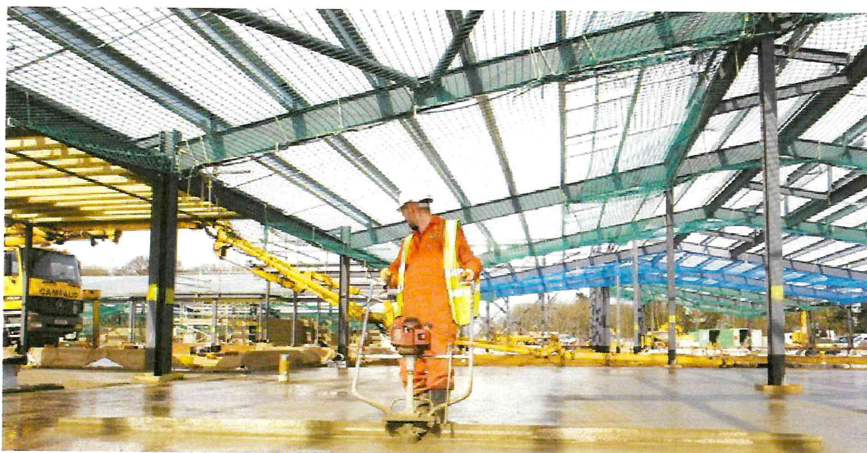
Safety nets installed before roof works start
