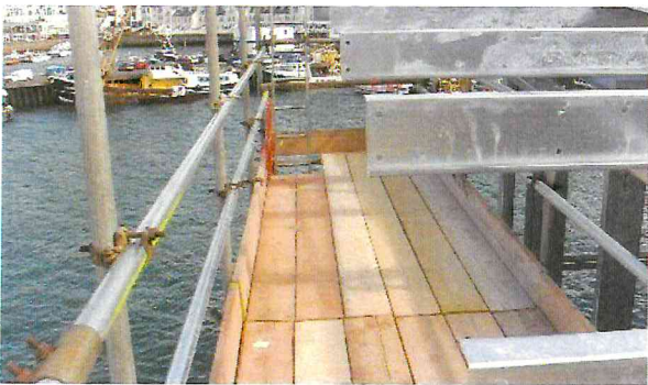
Objects protruding over a working platform present an impact or cutting hazard for workers on or moving across the platform
