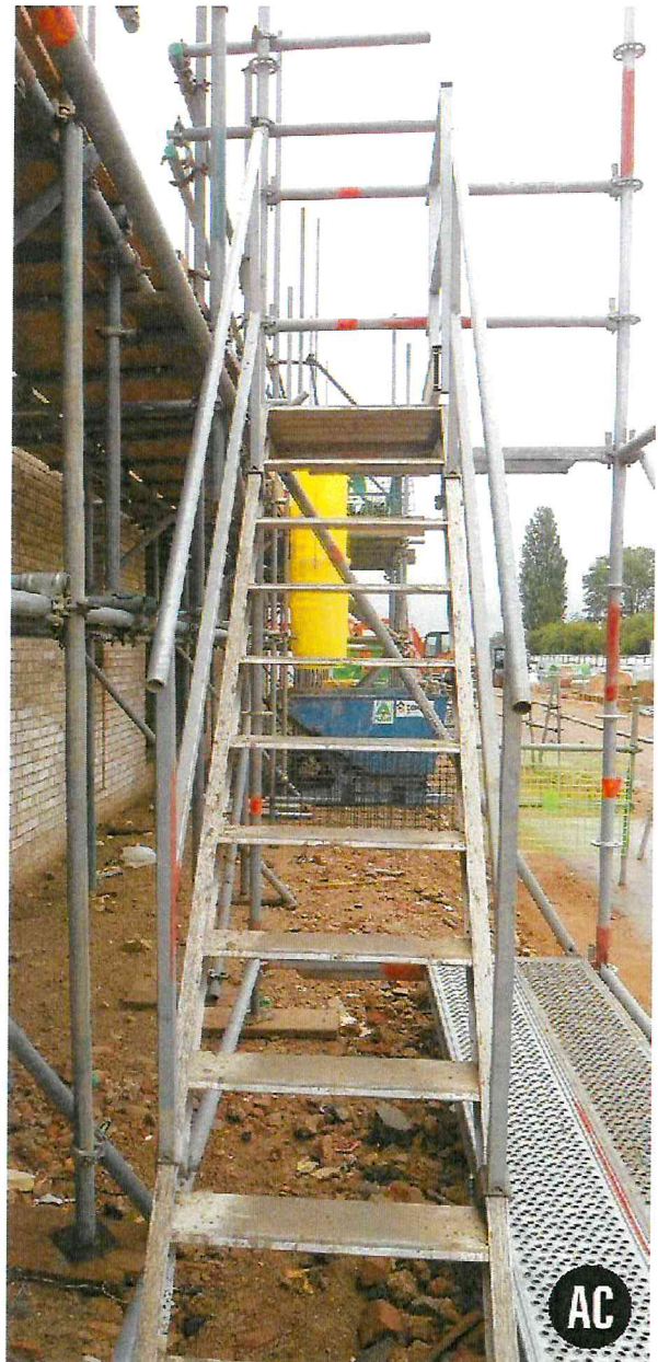
A purpose-built stair tower provides a safer means of access and egress
