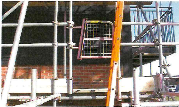
Ladder gates should be installed at all access points
