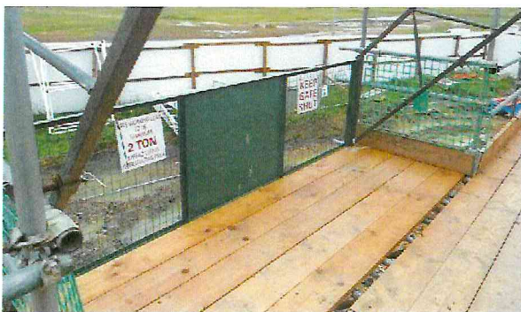
Loading bays should be marked with the rated capacity
