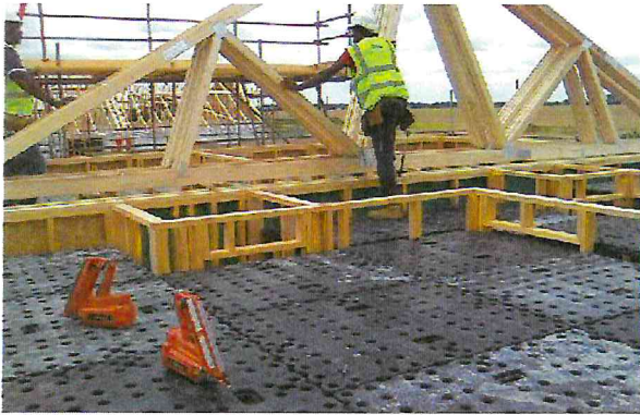
Proprietary decking system providing internal fall protection
