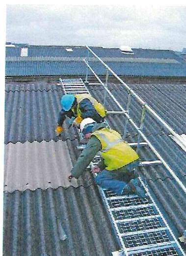
Examples of working at height activities with suitable control measures
