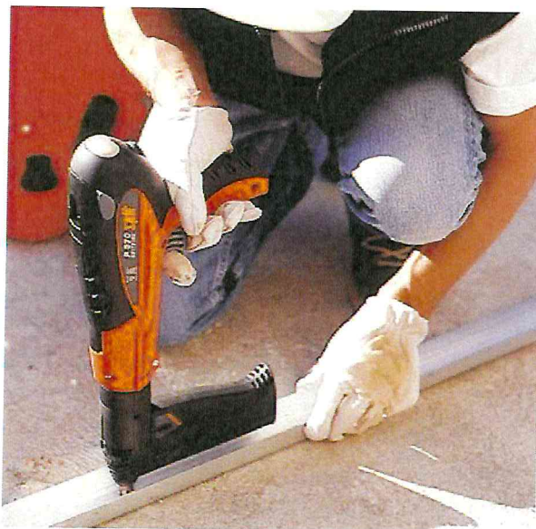
Using a cartridge tool on a stable surface
