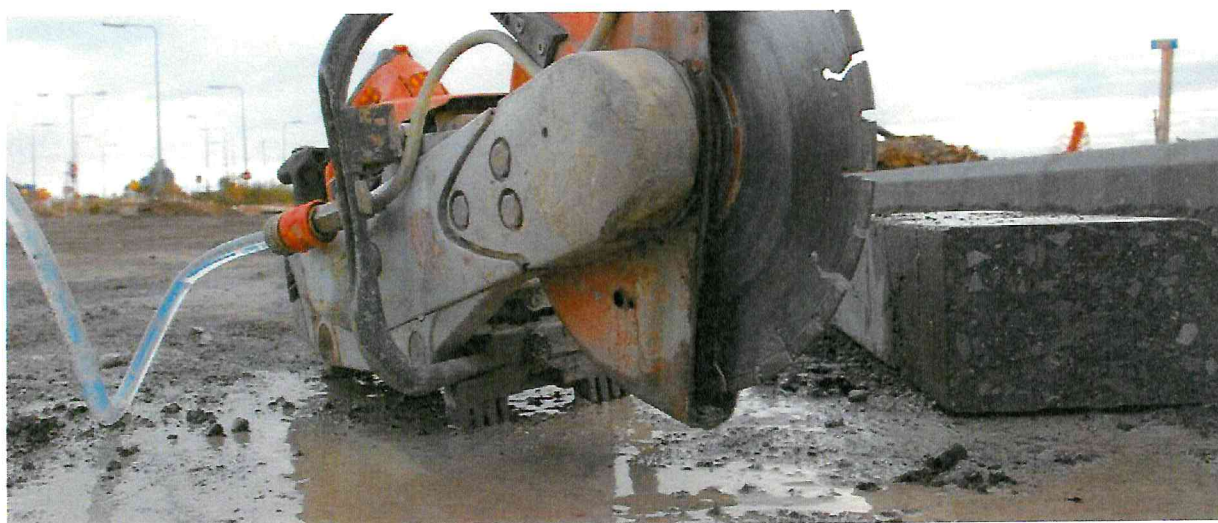
Dust suppression (wet-cutting) reduces exposure to silica and other harmful dusts
