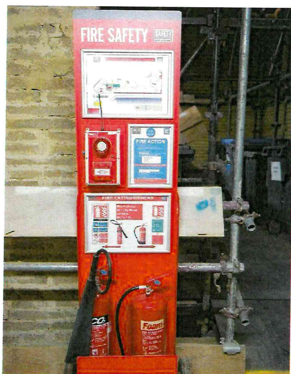
Example of a good fire point on site
