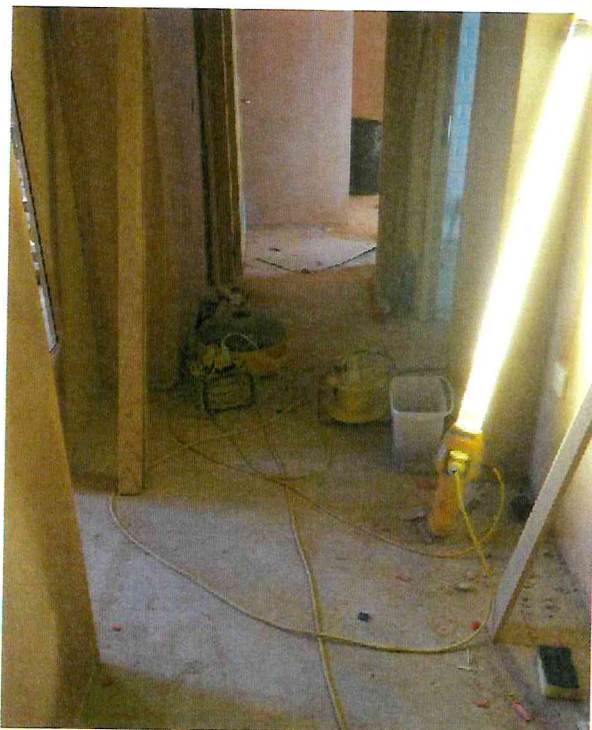
Poorly routed cables will increase the risk of damage and electrocution
