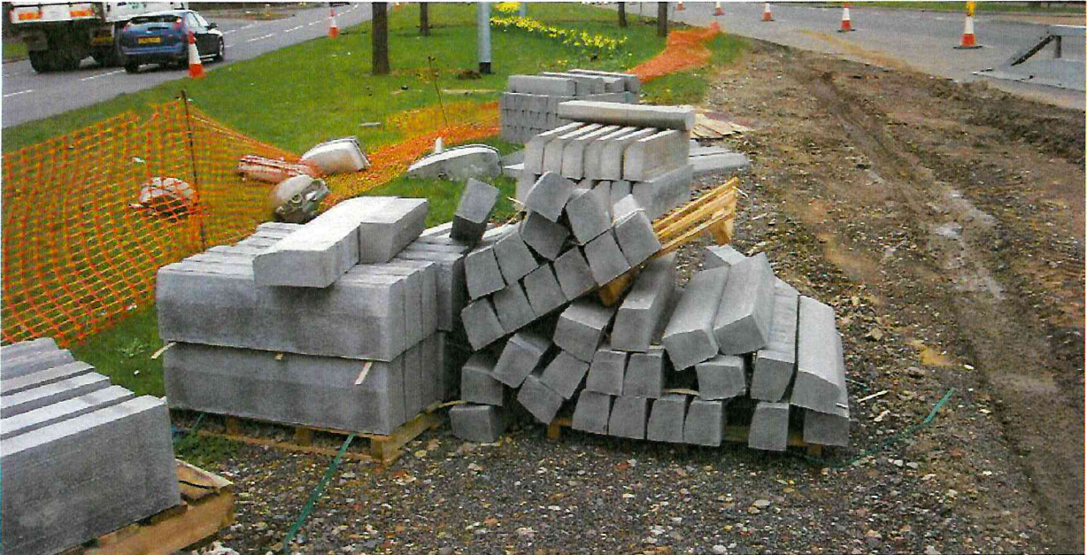
Always stack materials safely. This photo shows the results of bad practice
