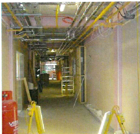
Examples of cables routed above head height to avoid tripping hazards
