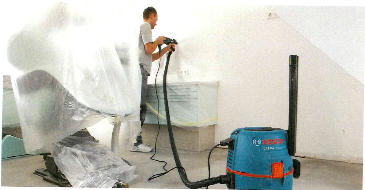
Drill with dust extraction
